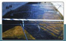
Sequential Batch Reactors have various locations that accumulate foreign materials. Foam and scum tend to collect in the pre-aeration zones while algae growth can become a problem in the EQ basin. The Eco-Blaster, BCS versatile mounting configurations can address these concerns. A buoyant mounting system will allow the Eco-Blaster, BCS to rise and lower with the liquid level to maintain control.
